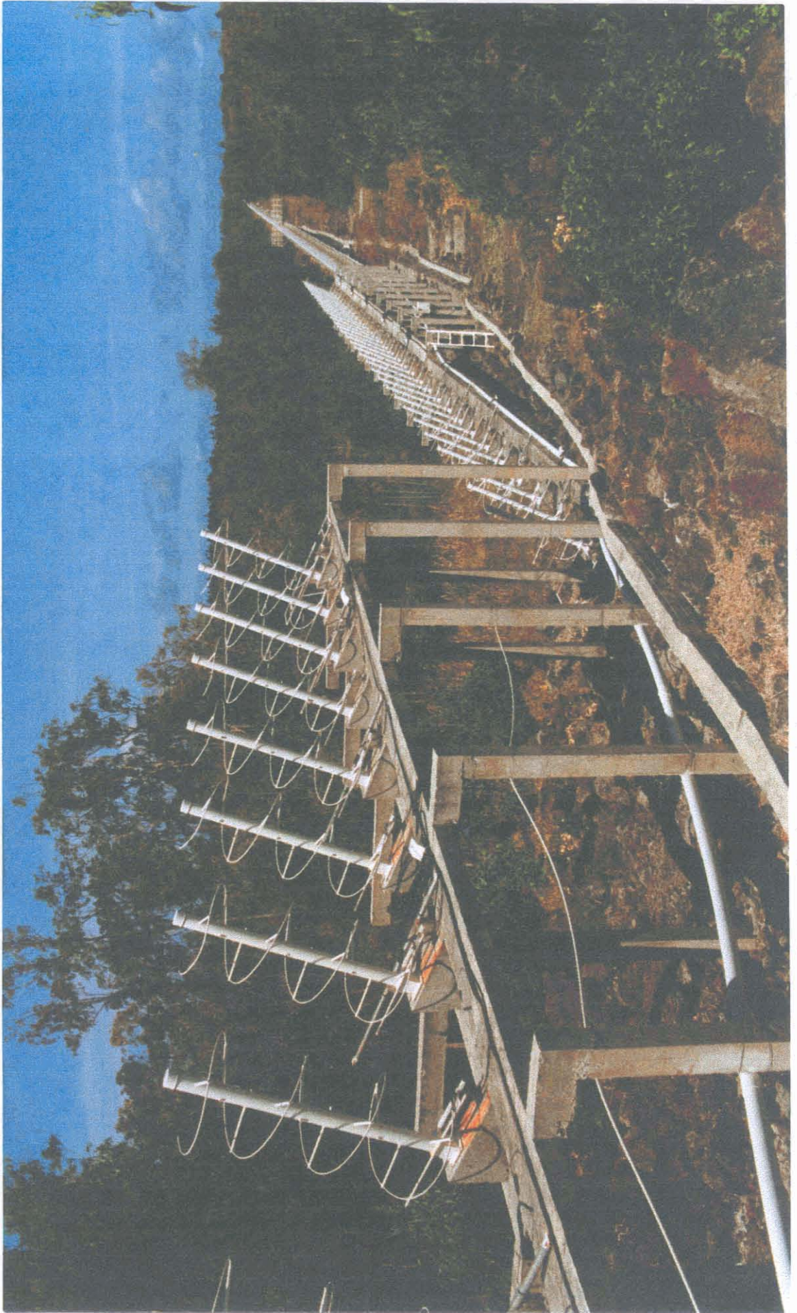
Figure 2.3: A view of the eastern arm. The non-coplanarity of the array is seen clearly.
