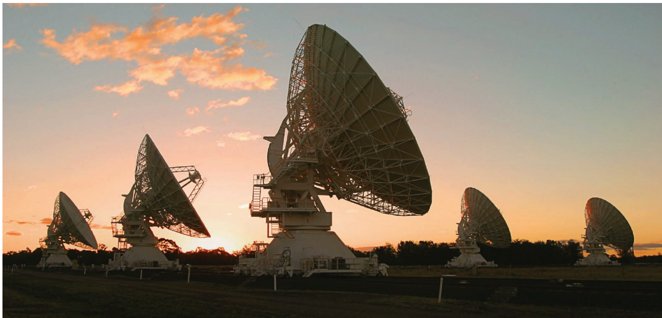
Figure 1. The ATCA, located at the Paul Wild Observatory near Narrabri, some 550 km north-west of Sydney. Displayed are five of the six 22-m Cassegrain antennas, here arranged in one of the hybrid configurations which include two antennas on the north–south spur. The latter was opened on 1998 November 26, just over 10 years after the ATCA opening on 1988 September 2.
